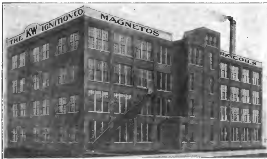
New factory of the K-W Ignition Company in Cleveland, Ohio.
